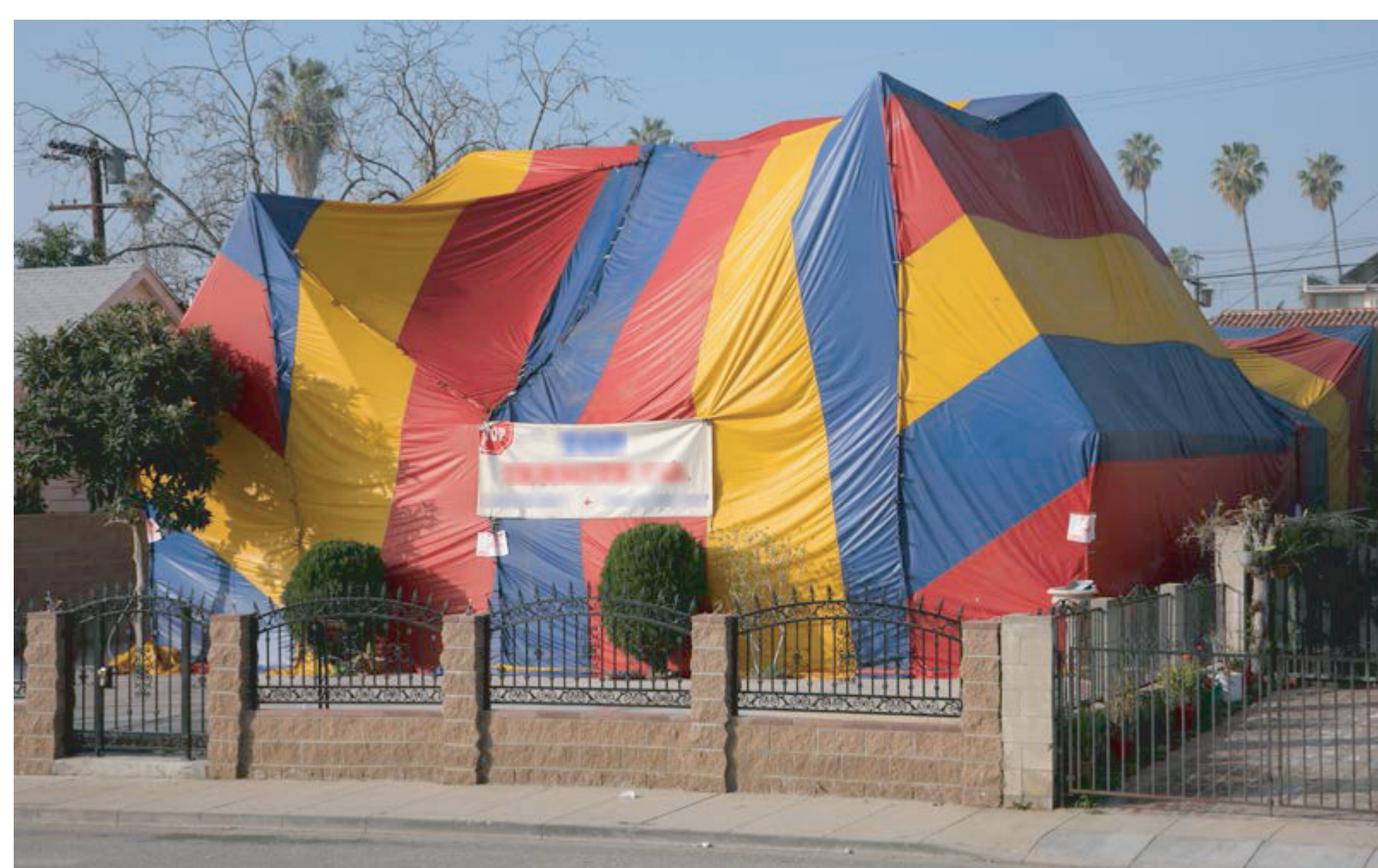
Figure 1: During structural fumigation, SO 2 F 2 is typically injected into a tented enclosure producing a toxic atmosphere of several parts per thousand that effectively permeates deeply into building materials over ~24 hours to reach the target pests (e.g., termites). SO 2 F 2 prevents insects from metabolizing the stored fats they need to maintain a sufficient source of energy for survival by disrupting the glycolysis cycle. Subsequent venting of the structure results in an estimated atmospheric emission of 88% of the injected amount.
